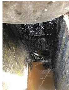
Figure 3-1. Photo of a catch basin polluted by an emulsifier product.
