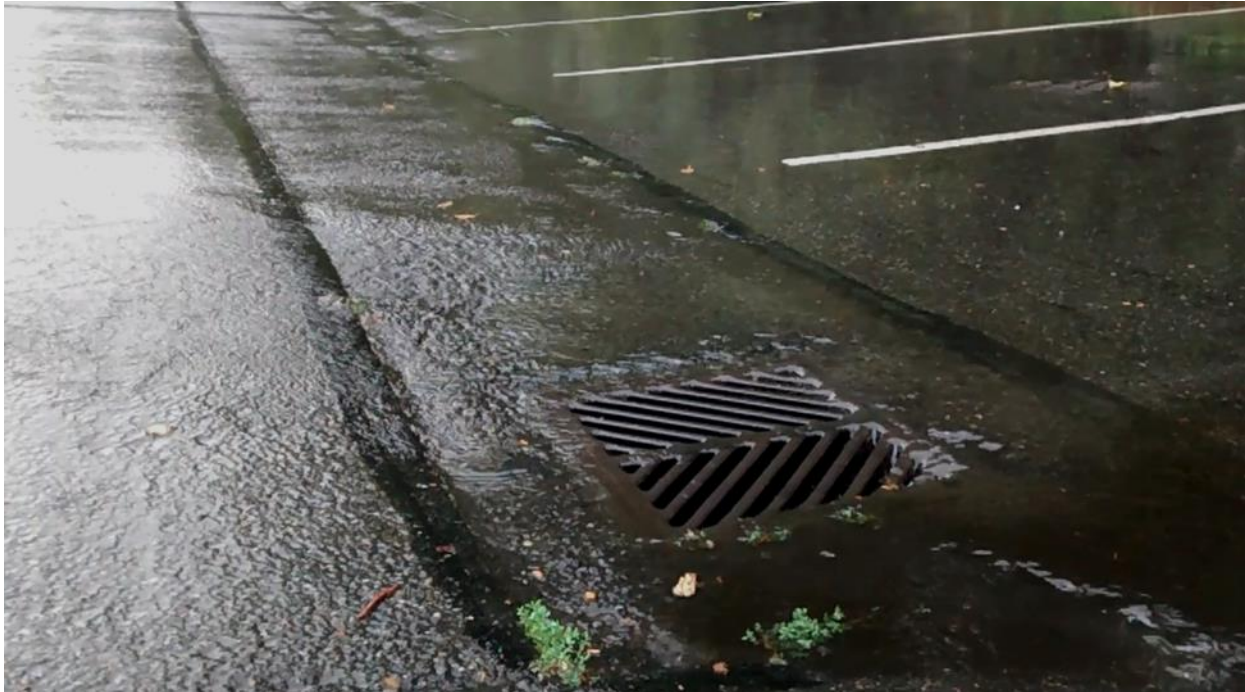
Figure 1-1. Stormwater runoff flowing into a storm drain before making its way to the Skagit River.
